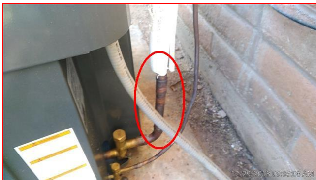
8.1 Missing Insulation
